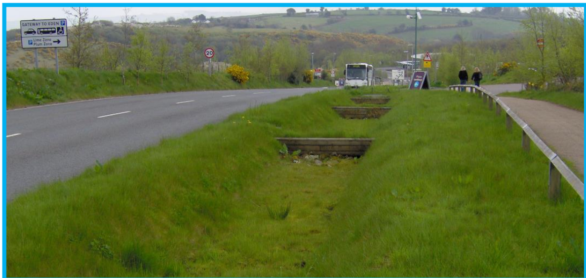
Fig 21 Typical swale with check dams – these can be earth and gravel dams to encourage attenuation, infiltration, evapotranspiration and evaporation (Eden Project).
