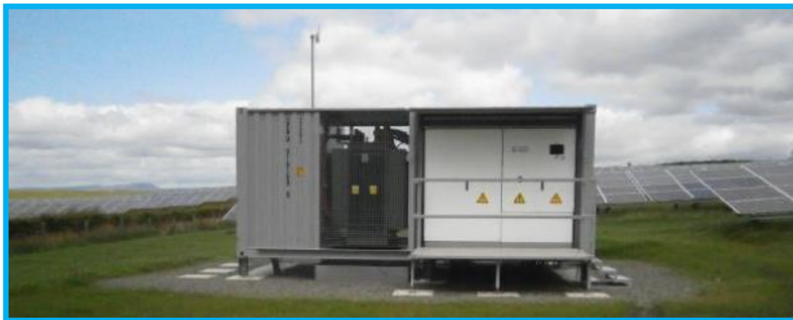
Fig 7 Typical containerised unit on pads over permeable gravel bed.
