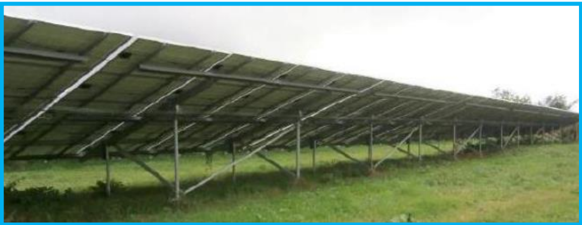
Fig 24 Avonmouth solar farm showing continuous vegetation under panels in a low-lying area. Note these arrays are only 450mm off the ground, reducing the light to the underside, but with no lack of flourishing vegetation.
